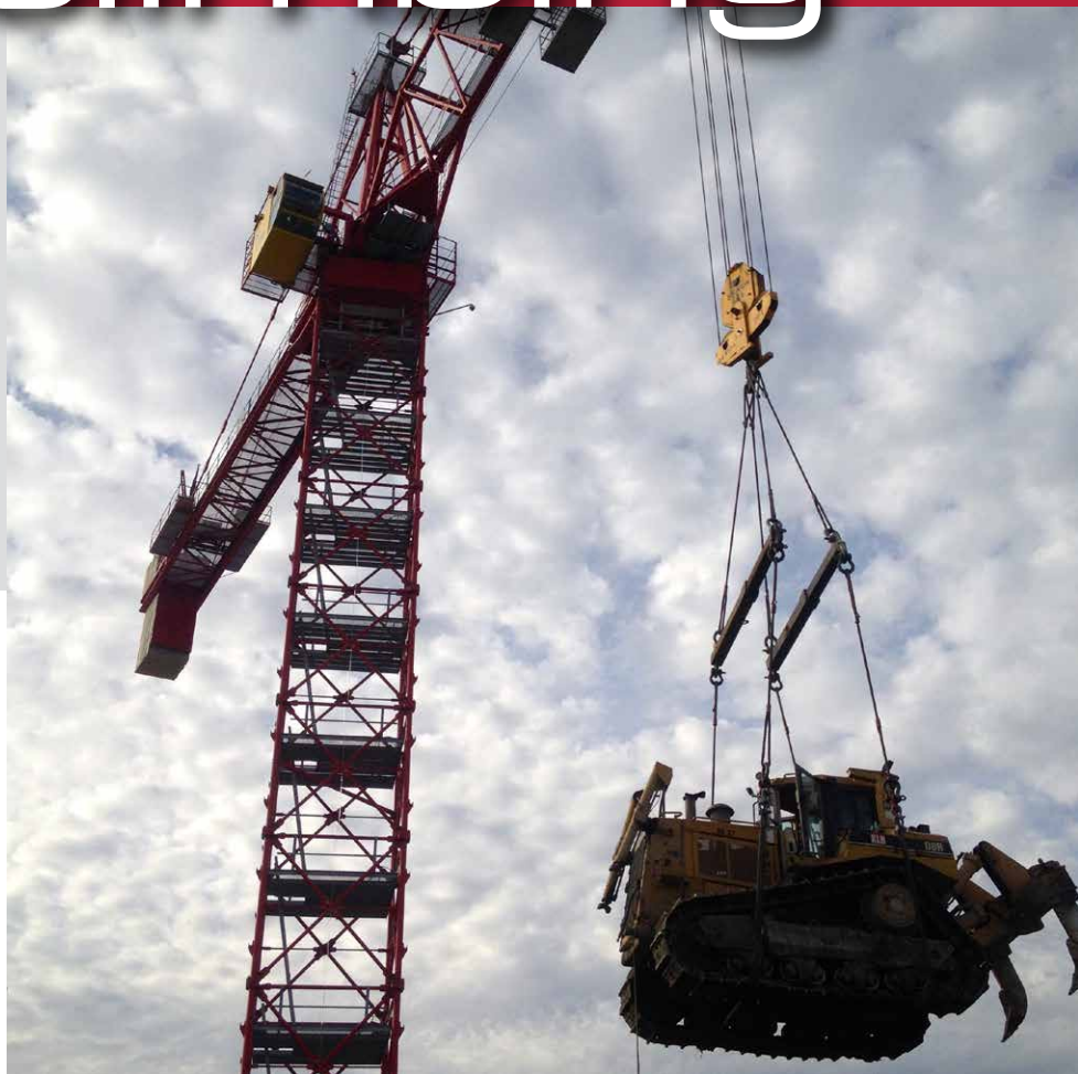
Jay Dee Contractors' custom-built Kroll K1800 lifts an 81,000-pound dozer.
